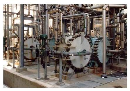
Fig. 4.153.: Sterilization station with spiral heat exchangers.
