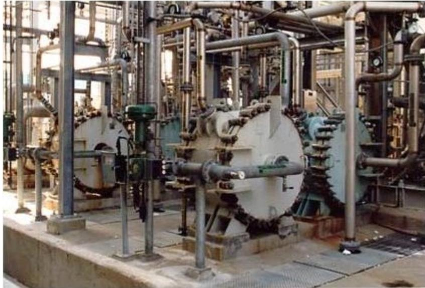
Fig. 4.153.: Sterilization station with spiral heat exchangers.
